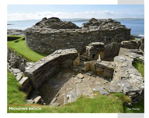
Damage has occurred from coastal erosion and the broch is now protected by a large sea wall. Built in the style known as 'cassying' it has resisted the Atlantic gales for decades.
