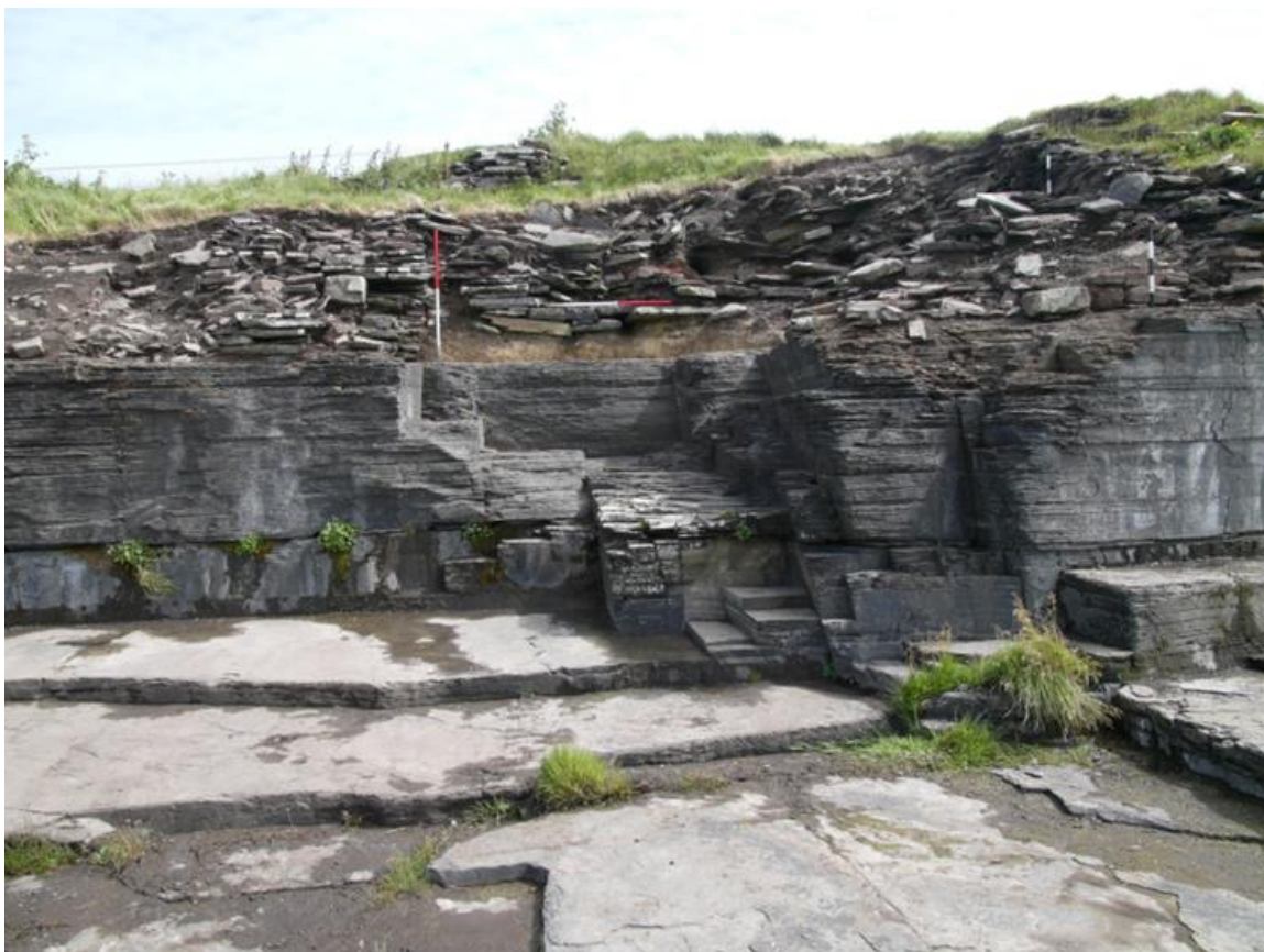
Fig. 3 South Howe: the later medieval or post medieval buildings eroding from the cliff face.
