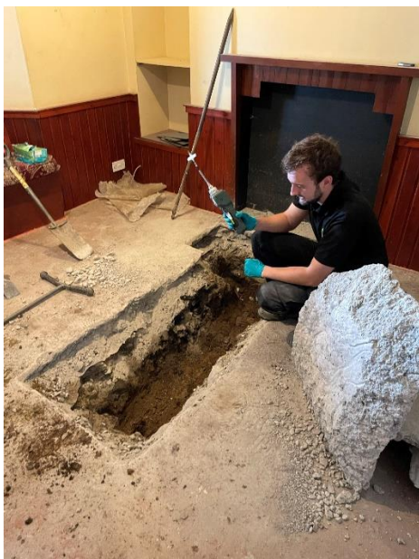
Remediation work at the Pier, soil testing and test hole drilling.
