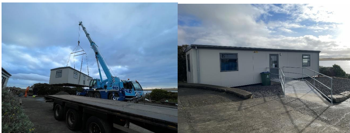
The cabin being delivered, and fully installed.
