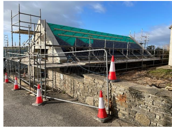
The building at the start of April 2024
